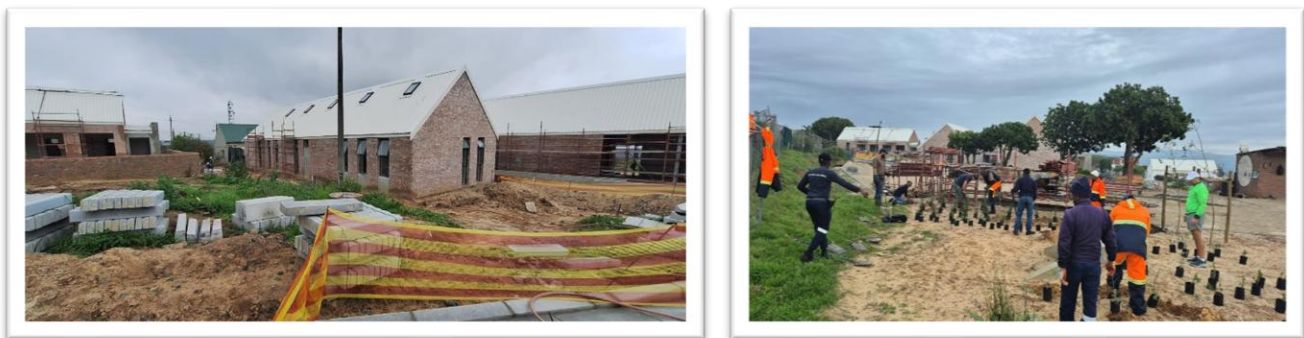
Figure 43: The upgrading of the visitor centre and administration complex at Bracken Nature Reserve.
